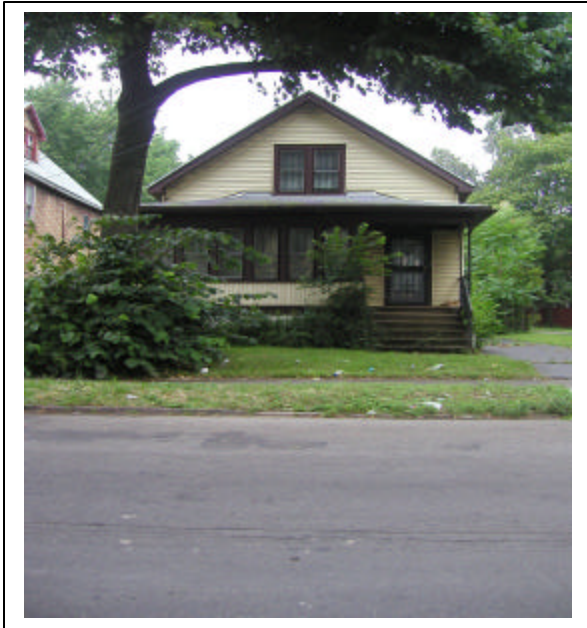
Photo 5: Housing Conditions in the Planning Area Two
