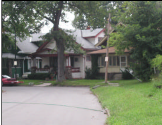
Photo 8: Typical Housing and Neighborhood Conditions
