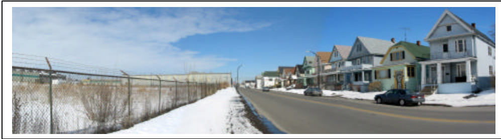
Photo 6: Grider Looking North toward East Delavan
