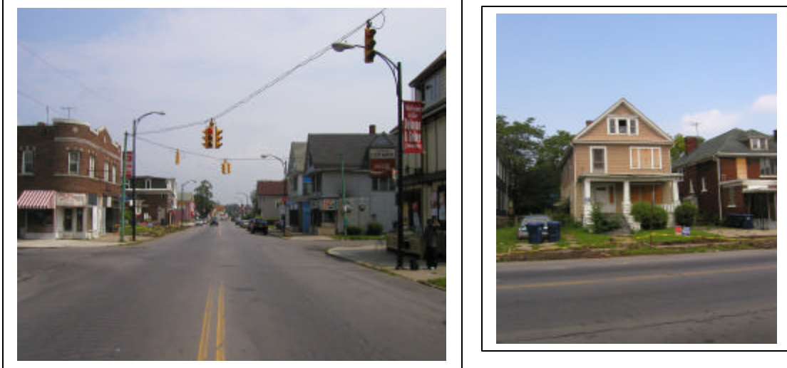
Figure 11: East Delavan Commercial Corridor
