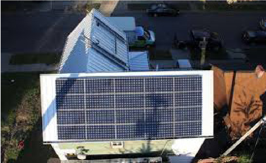
Solar Panels on Roof of Net Zero House (Photo from PUSH Buffalo)
