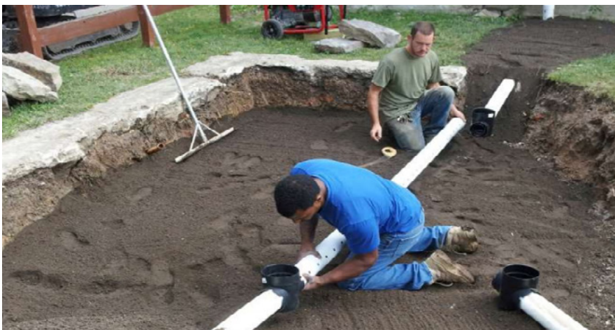
PUSH Blue Installing a Rain Garden (Photo from PUSH Buffalo)
