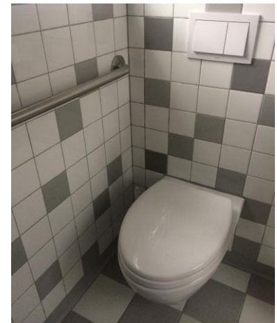
The grab bar extends the length of one wall, providing stability in the shower and doubling as a towel bar. The wall-mount toilet was expensive but worth it for the space savings in this tiny 3 1/2' x 5' bathroom.
