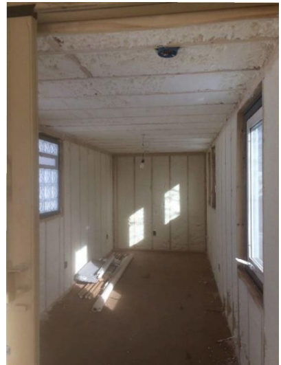
Portions of the framed-in interior, before, and after spray foam insulation.
