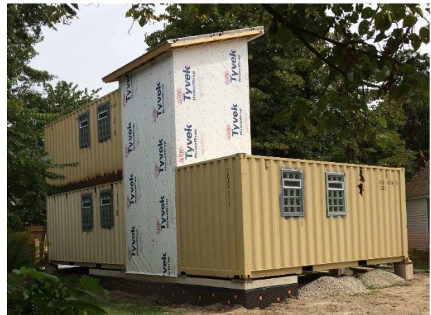
The conventional "stick built" portion went up quickly. It is a connector between the containers, allowing for our stairway to the second floor without having to cut into two containers.
