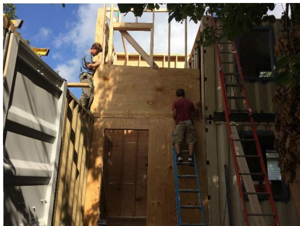
The conventional "stick built" portion went up quickly. It is a connector between the containers, allowing for our stairway to the second floor without having to cut into two containers.
